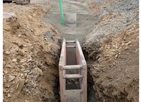
Installation of sanitary sewer pipe at manhole #22 (7/26/2021)
