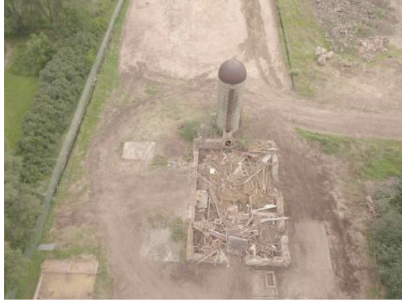
Remanence of the barn (7/20/2021)
