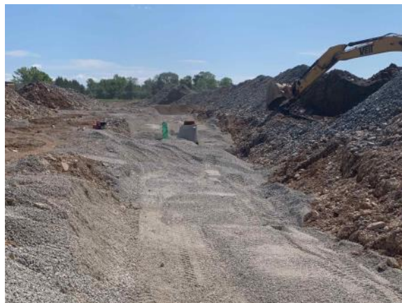
Sanitary sewer pipe installation looking East (7/30/2021)
