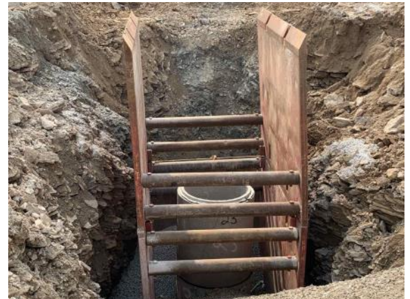
Manhole #23 being installed, near the soccer field (7/29/2021)
