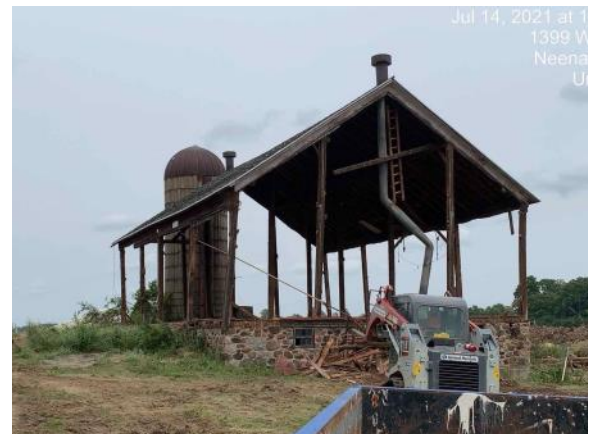
Still photo of the barn being demolished (7/14/2021)
