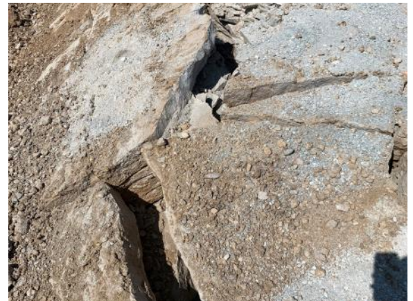
Fractured bedrock from blasting (7/30/2021)
