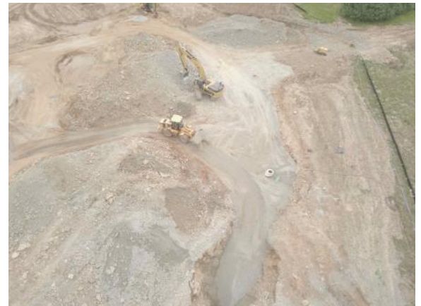
Aerial view of completed manhole #19 and #20, near the tennis courts (7/21/2021)
