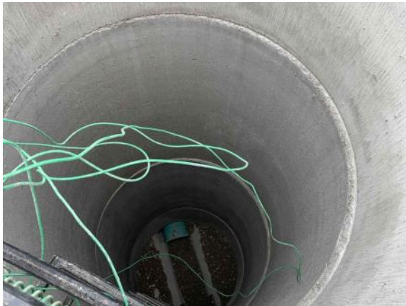
View looking inside the precast concrete sanitary manhole (7/26/2021)
