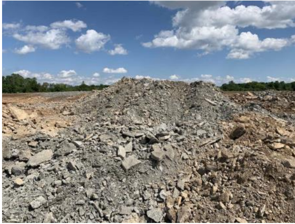
Large pile of stockpiled bedrock (7/1/2021)
