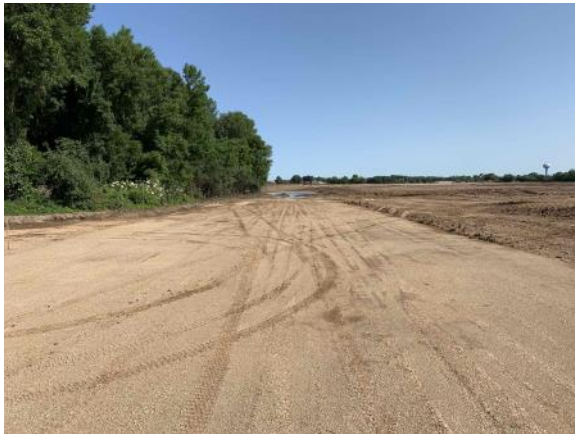
Future road on site is brought to sub-grade (7/2/2021)
